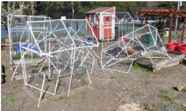
Vandals recently broke bird guards and PVC piping at the Miramonte garden. Photos Andy Scheck
